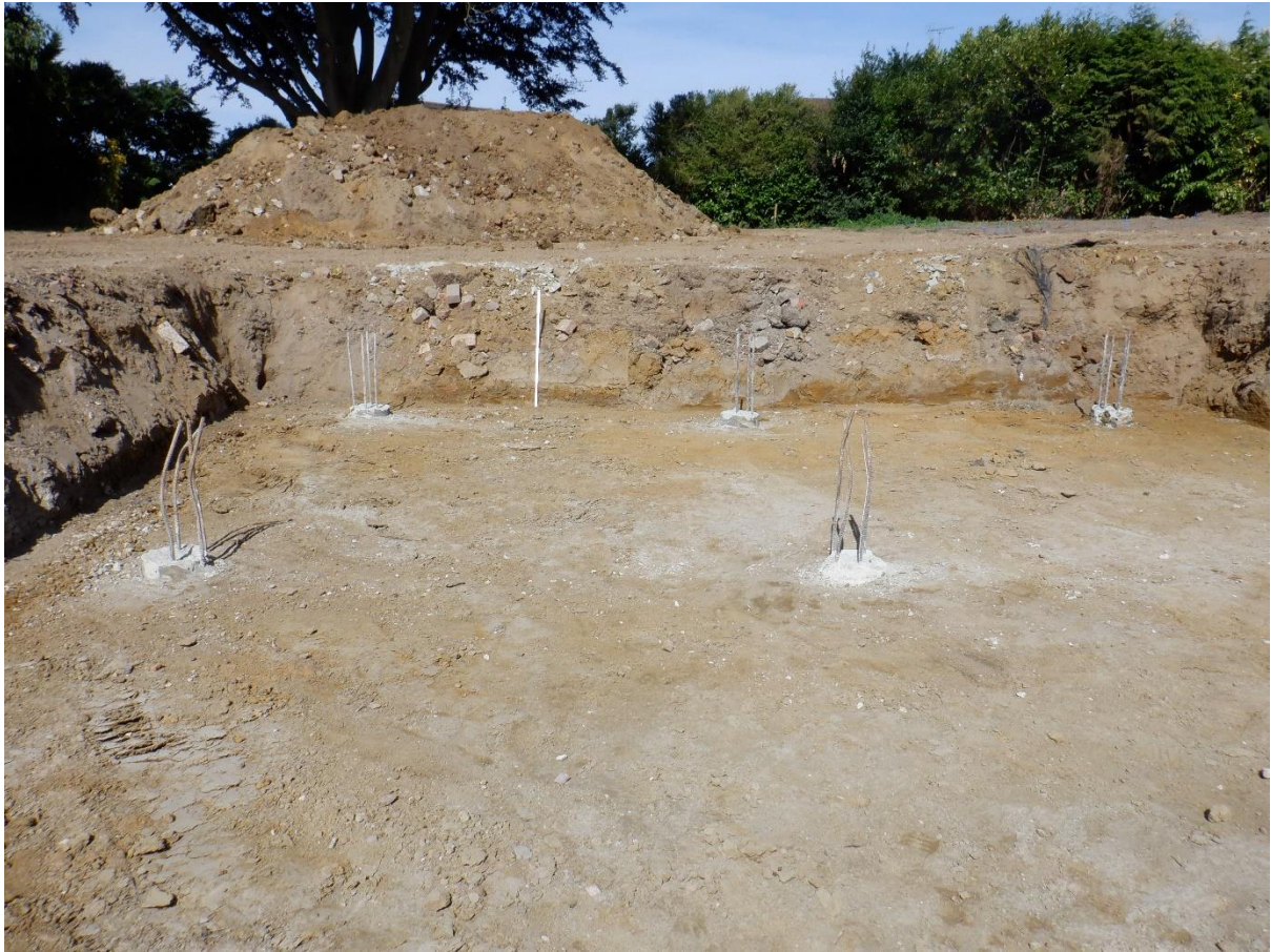
Plate 1. Setting out and ground reduction (looking North)
