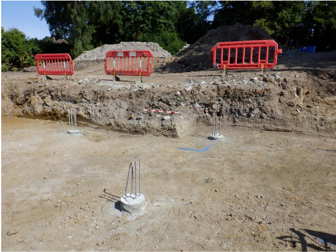
Plate 5. Foundation ground reduction (looking NE)
